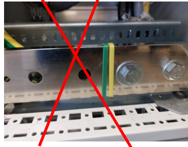
Shield bonding to the EMC shield busbar in the converter using an EMC shield clip
